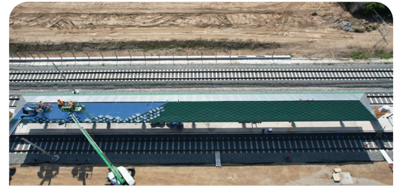
Crews installing metal roof for the future Glendora station.
