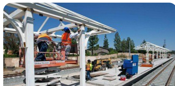
Crews preparing to paint the canopy frames their final color at the future San Dimas station.
