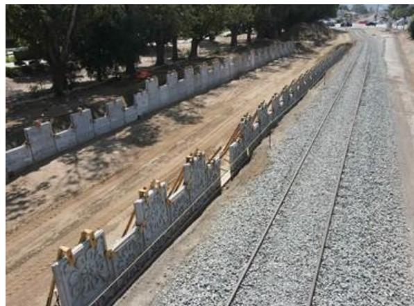
**Glendora Station Update:** At the site of the future Glendora station, crews have now completed the major structures for the pedestrian undercrossing that will provide riders access to the station platform. As seen in the photo below, the walls of the ramp to the station platform have been completed. Future riders will walk up this ramp - seeing the citrus design patterns on the walls - and onto the Glendora Station platform to board the trains.
