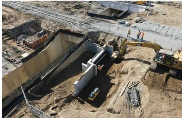
Elsewhere along the corridor, work is underway on the foundations for new bridge structures over Big Dalton Wash in Glendora, Puddingstone Channel and Live Oak Wash in La Verne, and Thompson Creek in Pomona. Two bridge structures will be built at each site - one for light rail, and one for freight - with the exception of Thompson Creek, which will only have a bridge structure for freight (under construction abutments for the Thompson Creek Bridge are shown in the photo above, right).
