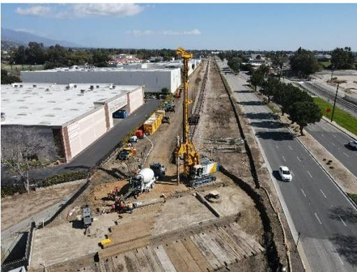
Photo(left): Crews are underway constructing the first bridges for the project. Two new light rail bridges and a freight bridge are being built over Puddingstone Channel in La Verne.
